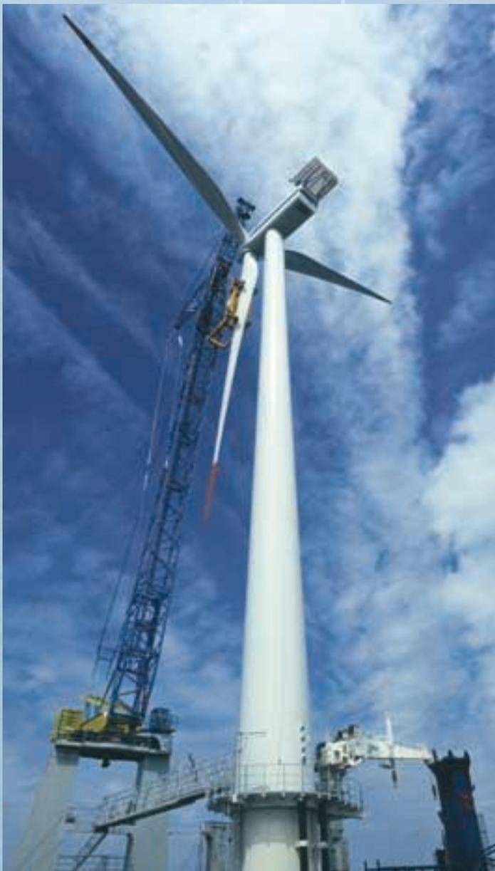
The wind turbines, each with a rotor diameter of 80 meters, are 110 meters tall. Each of the 450 tonne giants is supported on 25 to 40 meter long steel struts anchored deep in the sea bed. The wind power plant covers a total area of 20 square kilometers.
